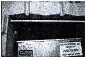
THIS SHOWS THE CHUTE LOCATION!
